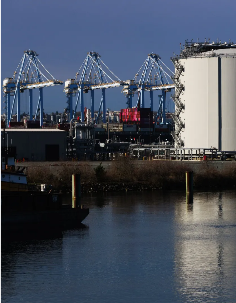
Pictured is Puget Sound Energy's liquefied natural gas facility at the Port of Tacoma. (Erika Schultz / The Seattle Times, 2024)
